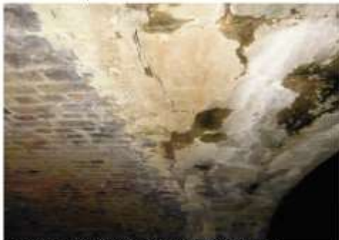
Photo 3: transverse and longitudinal fractures to soffits
